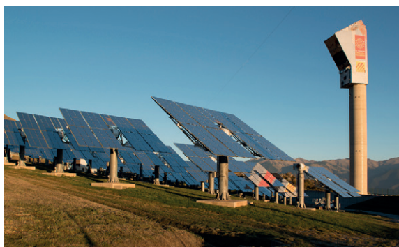
CNRS PROMES Thermodynamic solar power tower
