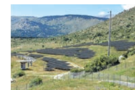
Engie Green Centrale solaire photovoltaïque bifacial
